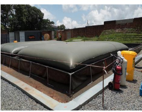
Project: Supply Fuel Storage Bladders with Spill Containment Berms
