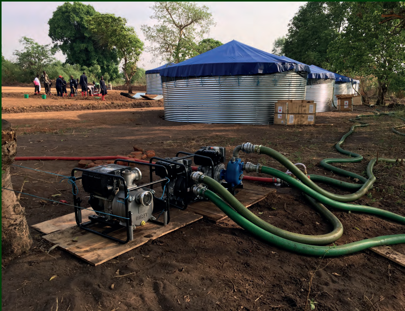
M40 Mass Sanitation Module Installation (Donated by Swedish Red Cross / Supplied by Butyl Products Ltd.) Uganda, 2017
